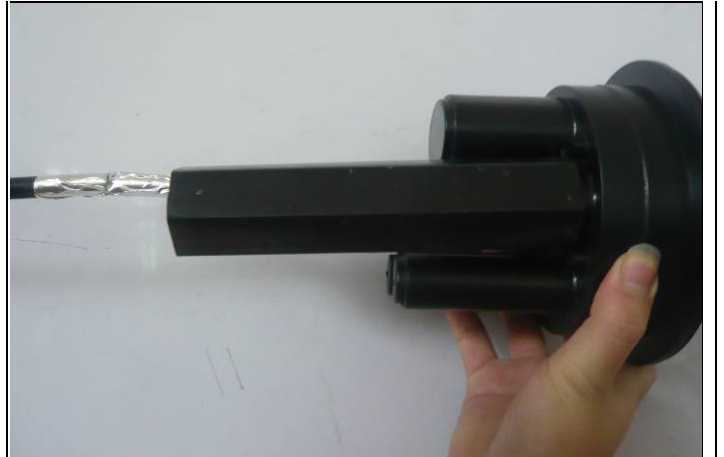
(11) Bound and even the heat-shrink part with aluminum paper to avoid burn caused by high temperature of blast burner.
